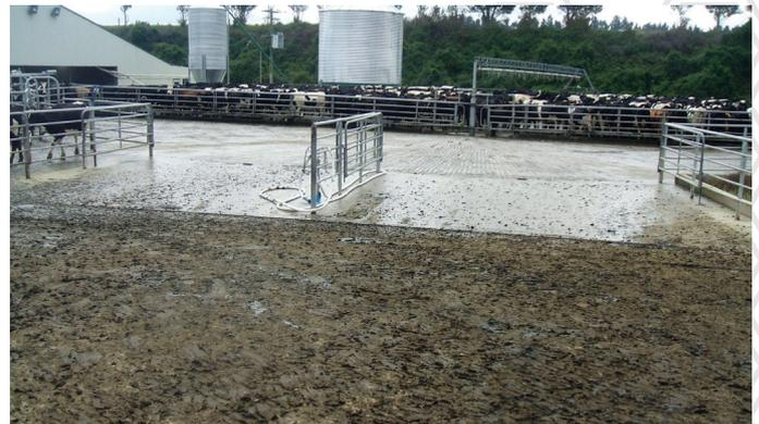
Entry to the milking shed showing a smooth & pothole free transition from race to concrete after 8 months usage.
