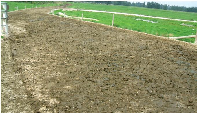
Race leading into the milking shed after 8 months usage. The soft metal is still in place & the integrity of the surface is preserved.
